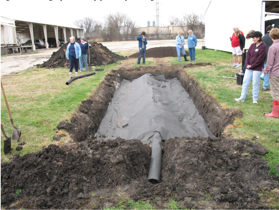
Figure 6. Placing the filter fabric
