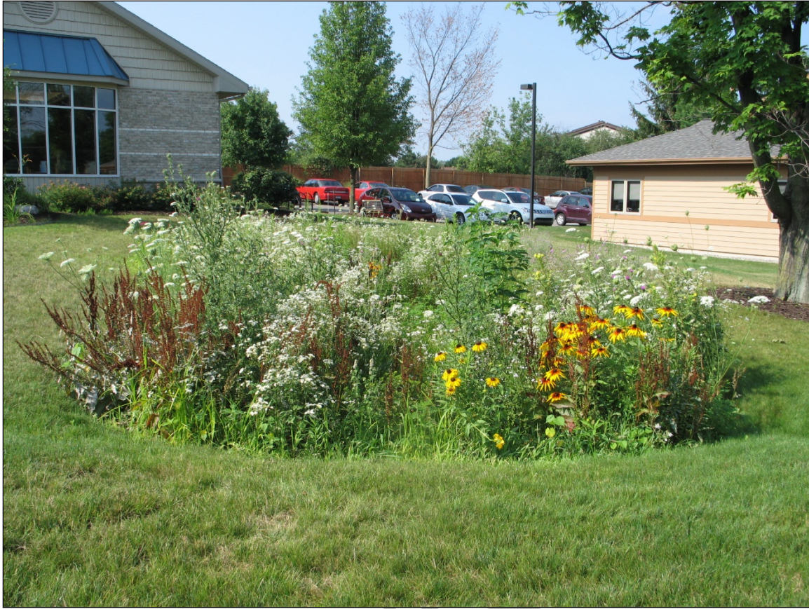
Figure 1. Rain garden built to capture rainwater off parking lot and roof
