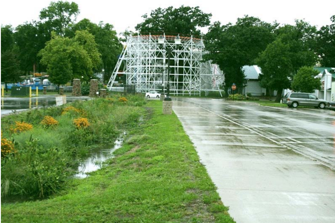
Figure 2. Rain garden built as an island in a retail parking lot (Courtesy of USDA, NRCS).
